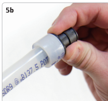
ProPEX Fitting Inserted into 1/2" Uponor PEX Tubing. Make the Fitting with a ProPEX Hand Expander Tool.
