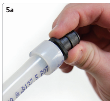
ProPEX Fitting Inserted into 1/2" Uponor PEX Tubing. Make the Fitting with a ProPEX Hand Expander Tool.
